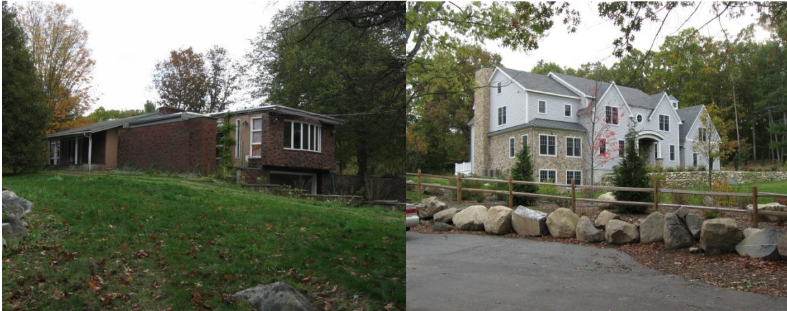
Residences at 16 and 22 Bypass Road
